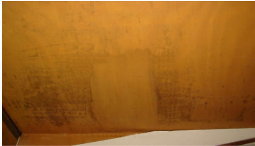
Typical example of surface mould
